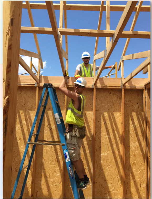
▲ Donning hard hats and tool belts, the team help builds a home beam by beam.
