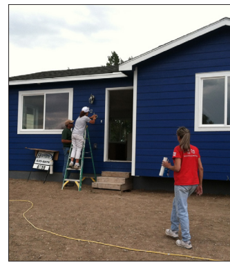
Lynda Zeringue installs house numbers on new Habitat for Humanity home.
