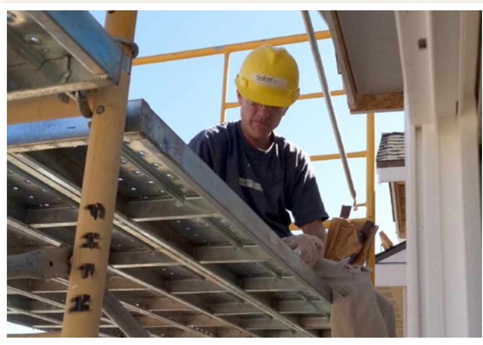
SCOTT HAVLICK INSTALLED SIDING ON A HOME AS PART OF THE FLATIRONS HABITAT FOR HUMANITY PROJECT.
