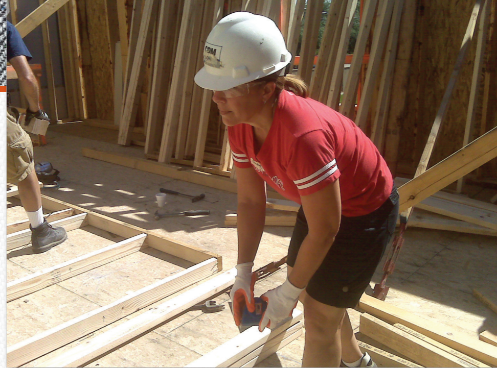
Sandy Thoele builds a wall for a Habitat for Humanity home.
